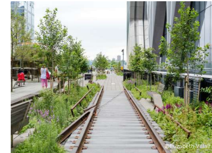
Joshua David and Robert Hammond founded Friends of the High Line, to advocate for the reuse of a disused railway line as a public space.
